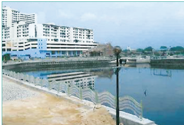
Fig. 1: Picture of S10 flood mitigation holding pond in Penang.
