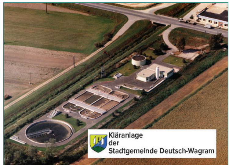
Fig.1: Wastewater Plant at Deutsch-Wagram
