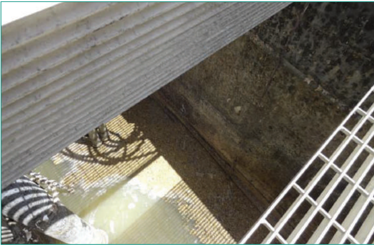
Fig. 5 & 6 These pictures further demonstrate the lack of new buildup of the grease cap when seen from a side view and through the grate from the top.
