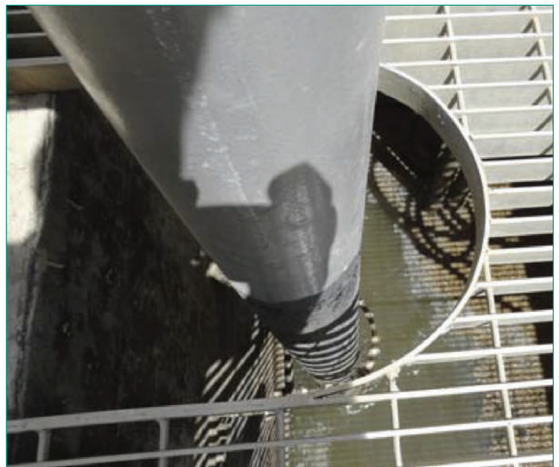
Fig. 5 & 6 These pictures further demonstrate the lack of new buildup of the grease cap when seen from a side view and through the grate from the top.
