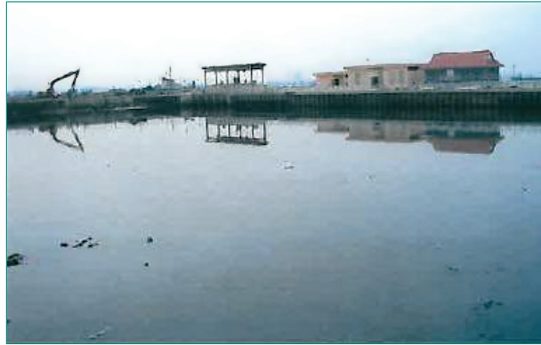
Fig. 2 & 3: Additional pictures of the pond and drainage system.
