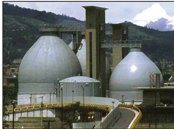
Typical industrial wastewater digester
