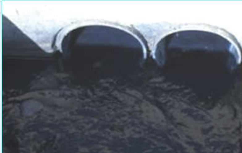
Fig. 2: The effluent from the plant shows extreme level of indigo pigment in the wastewater.
