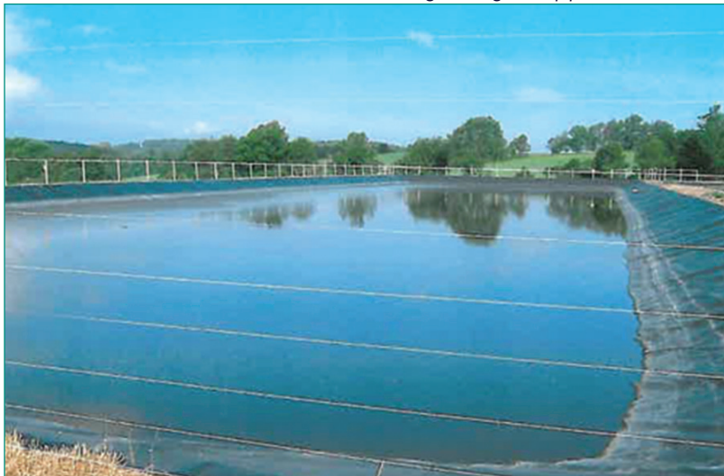
Fig. 3: The second lagoon was completely cleared of solids after the six-month pit treatment.
